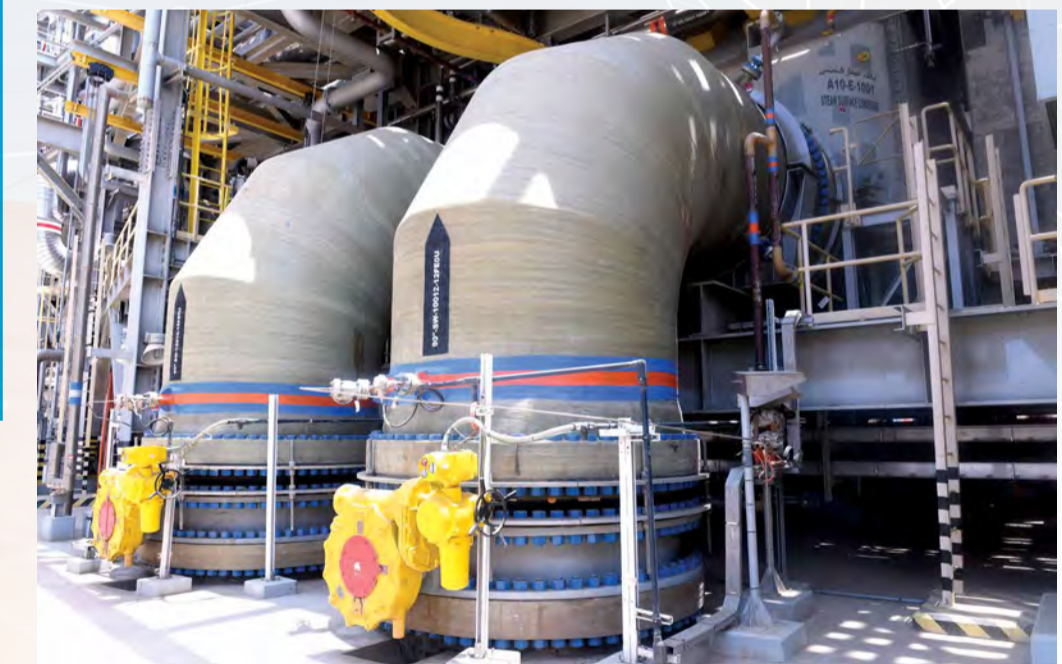
Nonmetallic piping at Jazan Refinery Complex.
