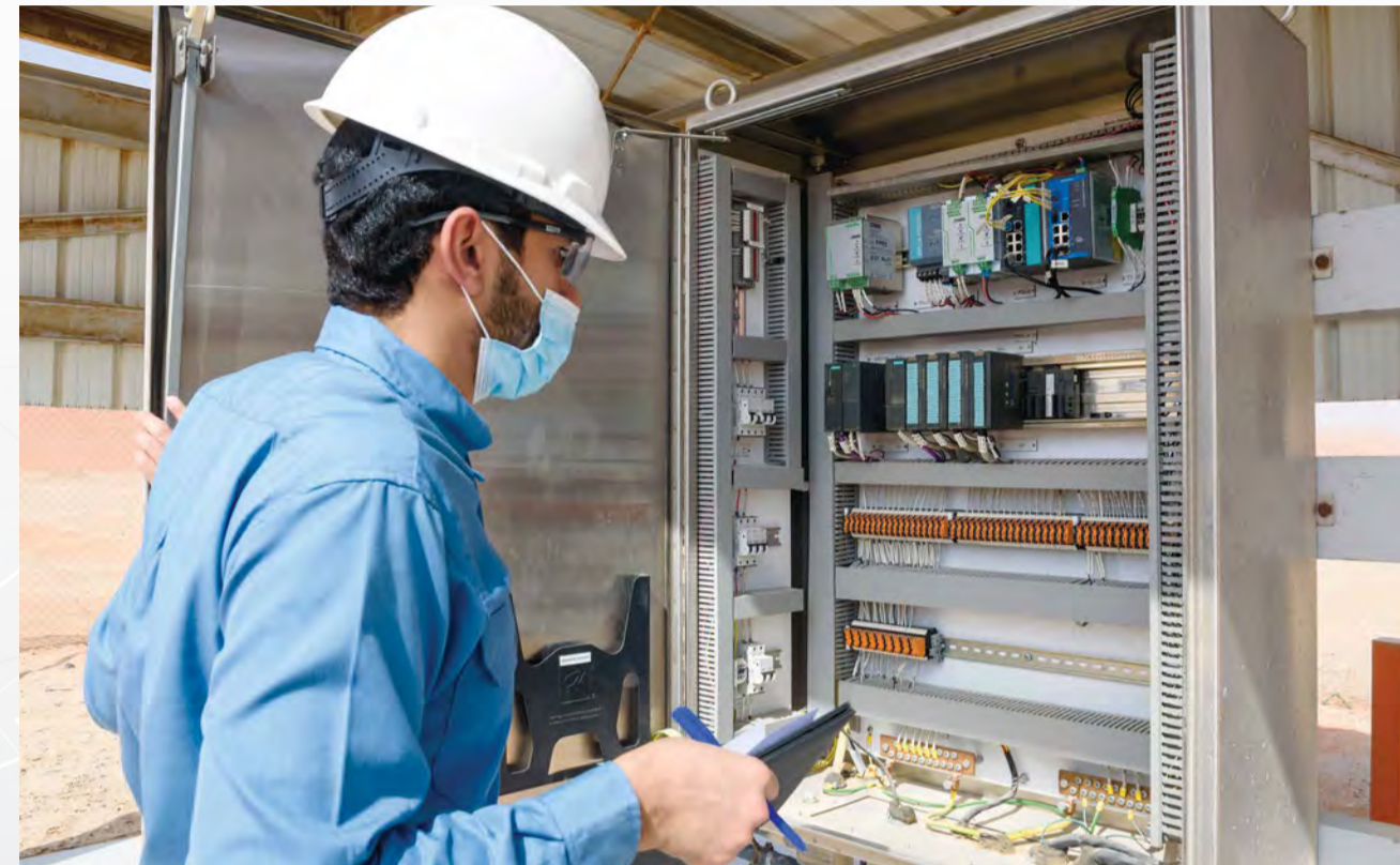
At a Shaybah pipeline junction, field operator Abdullah R. Fadly checks equipment powered by solar panels.
