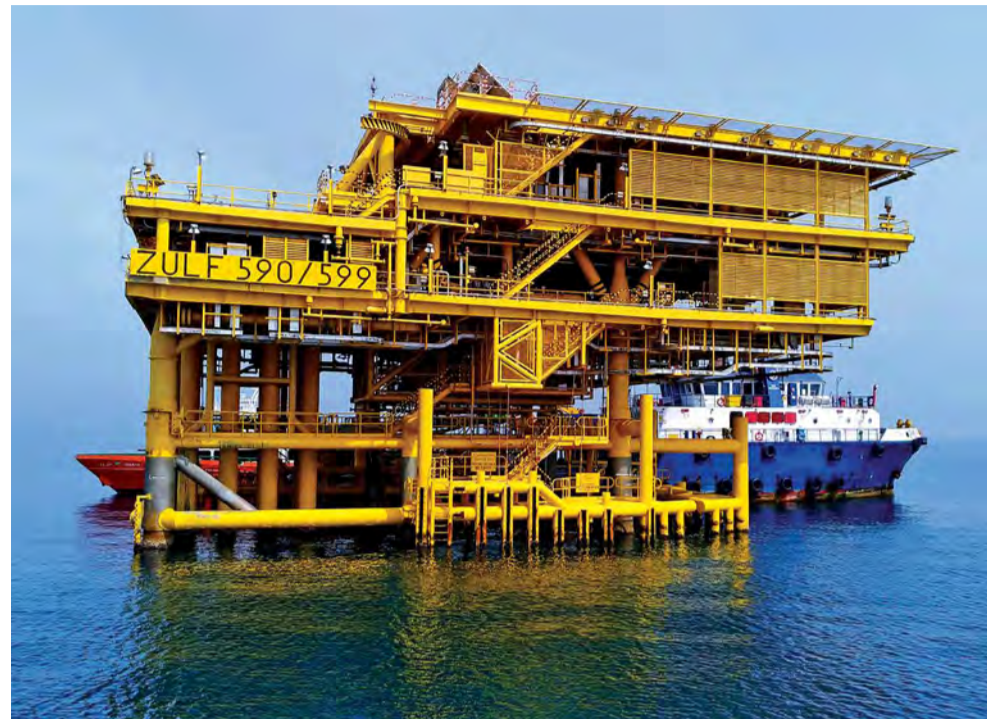
Design facilitates the circular economy and Aramco has a standard offshore wellhead design that can be used again and again without replication of engineering.
