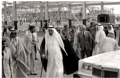
Berri Gas Plant, inaugurated in 1977 by King Khalid bin Abdulaziz Al Saud, was the first Master Gas System facility.
