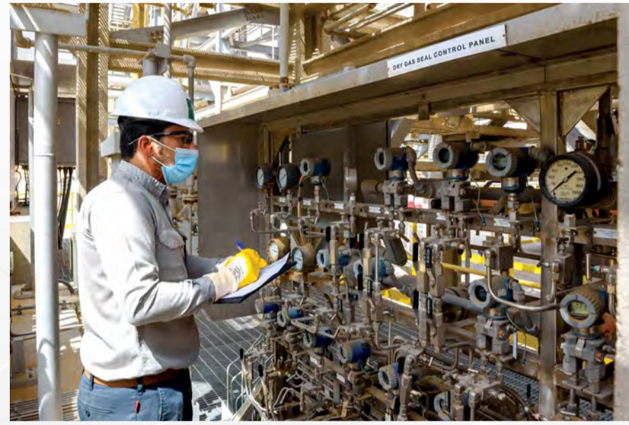
Yasser Y. Hakami, checking gas compressor readings at a Shaybah GOSP, says taking care of the plant’s equipment is an important part of his life. “I will be sad if anything happens to the equipment,” said the foreman, who received his Aramco apprenticeship training in ‘Udhailiyah, Ras Tanura, and Tanajib.
