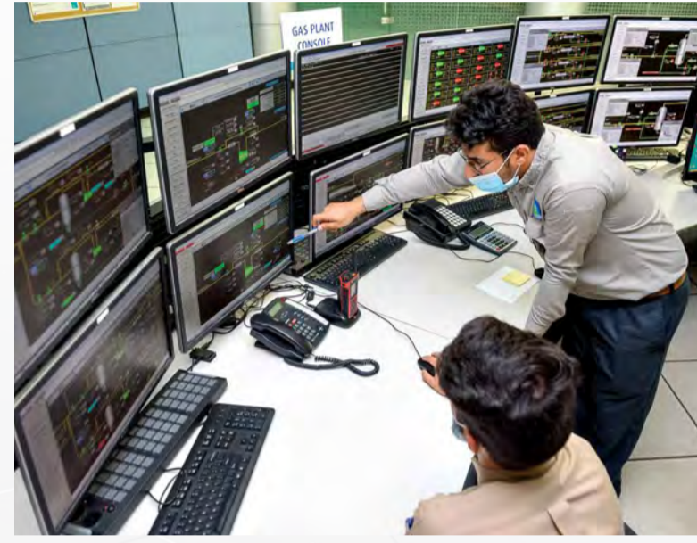
Aramco’s GOSPs integrate real-time data into the production processes, and inside a Shaybah central control room, console operator Badr M. Almutairi and foreman Yasser Y. Hakami keep a finger on the plant’s pulse by assessing operational monitoring information received by the nerve center from the gas compressor.
