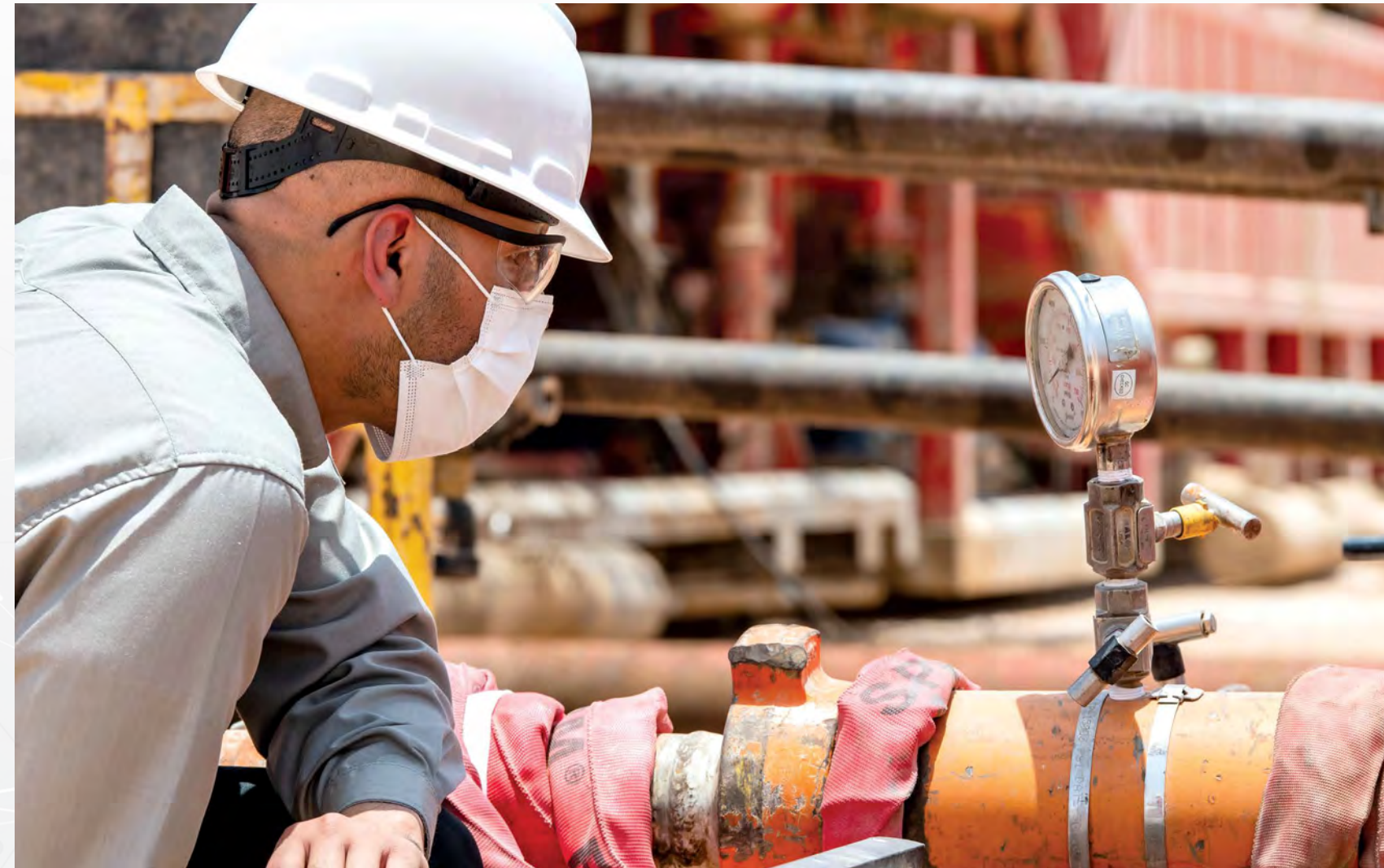
Foreman Saad S. Garni monitors the successful connection of a gas tie-in from drilling rig ADC-45 to the wellsite's production manifold flow line.
