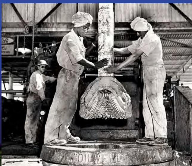
In this photo from 1949, two Saudi employees of Aramco guide a drilling pipe and bit through a rotary table on a rig near Abqaiq. Today, the scope of drilling is similar, although more advanced. Photo by T.F. Walters.
