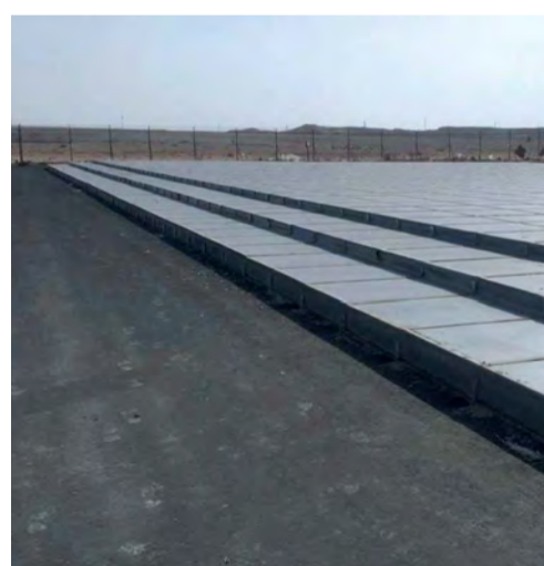
Located at the end of the runway, the EMAS aviation safety system is a breakable cement. The cement will crumble when an airplane runs over it, thereby preventing the aircraft from overrunning the end of the runway and causing an accident.
