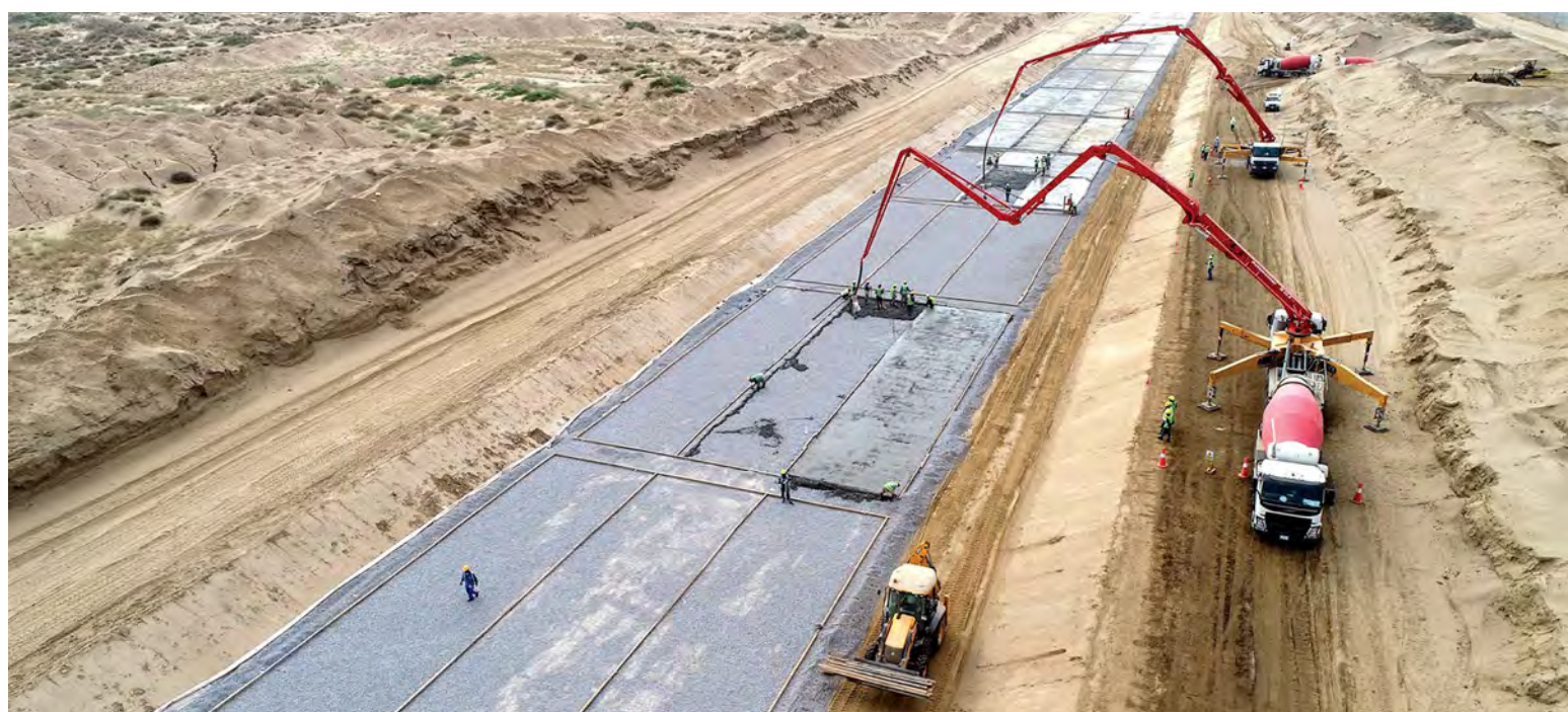
Nonmetallic solutions have been deployed successfully at Jazan operations, including using glass fiber reinforced polymers bars for a 20-km concrete flood mitigation channel.
