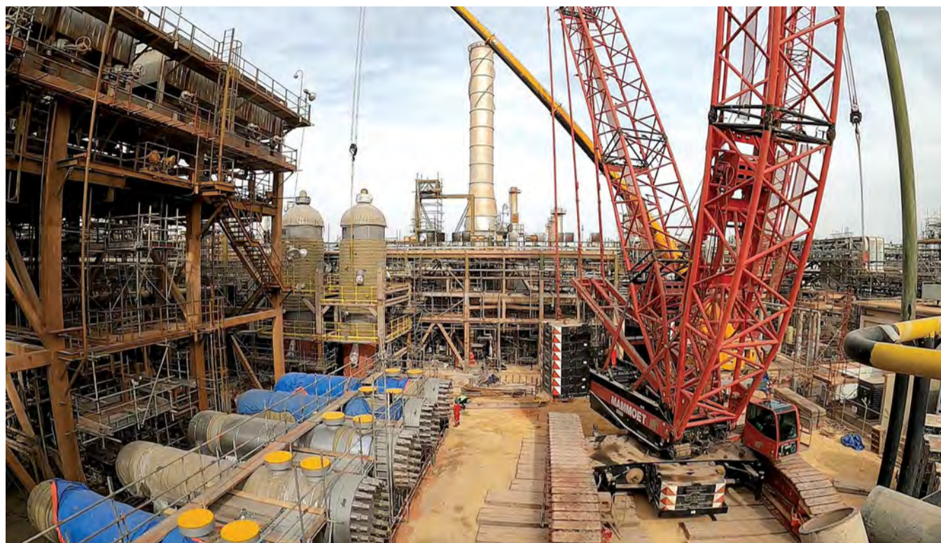
The installation of two new platformer heat exchangers being lifted in place with an 800-ton capacity crane during the Riyadh Refinery upgrade.
