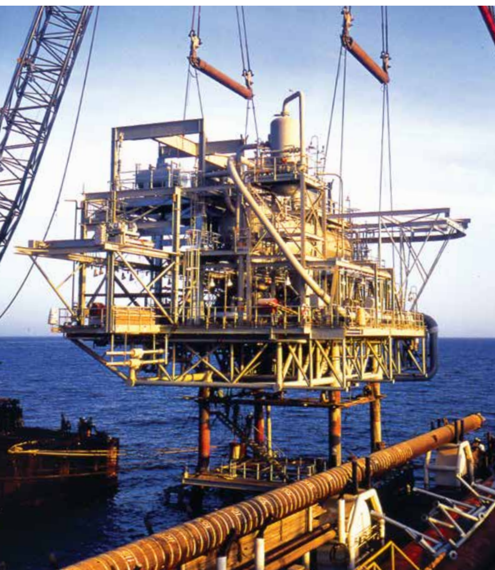
A gas-oil separation plant (GOSP) is lifted into position in the Marjan offshore oil field in 1973, part of Aramco's capital projects program that increased offshore oil processing capacity by 1 million bpd. In addition, eight onshore GOSPs, with a combined capacity of more than 2 million bpd, were constructed in the first nine months of the year.
