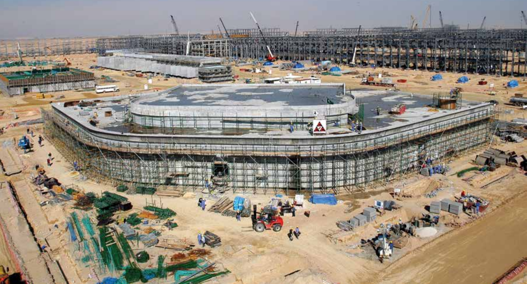
The massive Khursaniyah oil- and gas-processing complex, shown here during construction, was built to process 500,000 bpd of Arabian Light crude oil and 1 billion scfd of associated gas.
