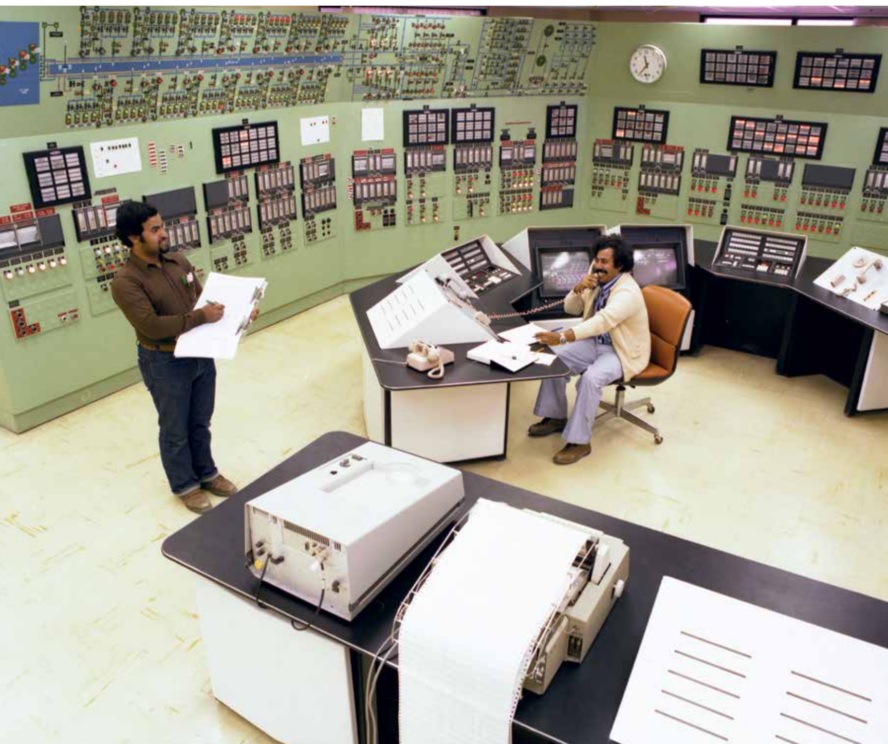
Operators in the control room of the Qurayyah Seawater Treatment Plant in 1979 monitor the processing and delivery of 4.2 million bpd of seawater for injection into oil fields to maintain reservoir pressure.
