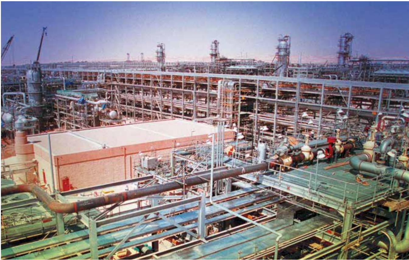
Hawiyah Gas Plant, shown here under construction in 2001, was designed to process 1.4 billion standard cubic feet of nonassociated gas per day for the Master Gas System. Aramco entered the new century with an increased emphasis on production of natural gas to fuel the Kingdom's economic diversification plans.
