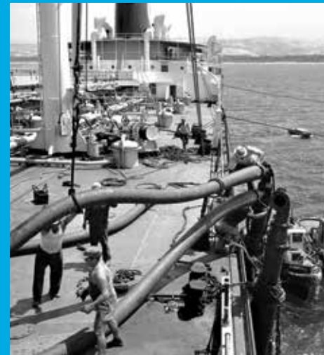
A combined crew of Tapline and oil tanker personnel hoist submarine crude oil loading lines aboard ship in July 1961, an action repeated thousands of times over the life of the Tapline terminal at Sidon, Lebanon.
