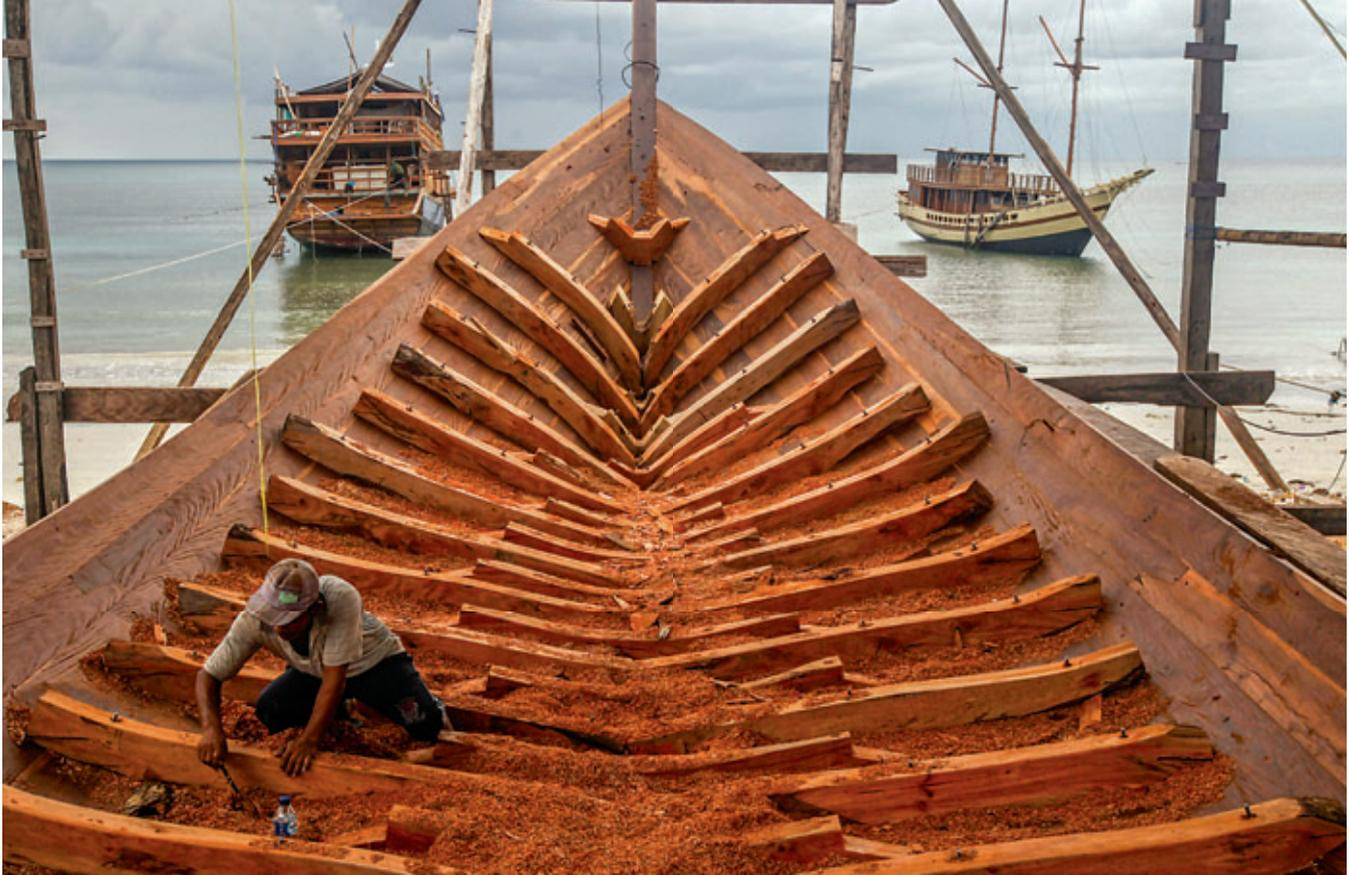
A craftsman scrapes sawdust where ribs meet hull planks on a *pinisi* boat under construction in Tanah Beru, where Haji Abdul Wahab, **RIGHT**, has been building the iconic Indonesian schooners for more than 30 years.
