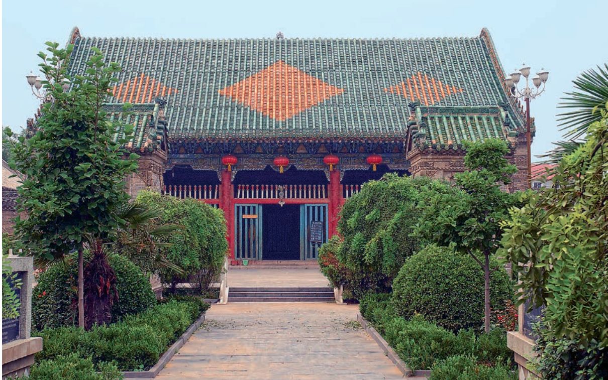
A rectangular, wooden post-and-beam structure raised on a platform with outer walls of brick and a tile roof, the Zhuxian Mosque in Kaifeng, Henan province, above, differs little from the worship hall at the Buddhist monastery at Ledu, on the Tibetan Plateau near Xining, left. At the mosque, the two small pavilions on either side of the path—which in a Buddhist setting might be drum and bell towers—here contain stelae, or upright stone slabs, chronicling the history of the mosque.
